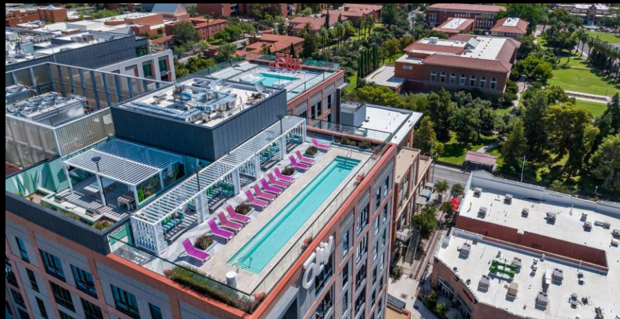
Cimarron Circle Construction, Oliv Spa
