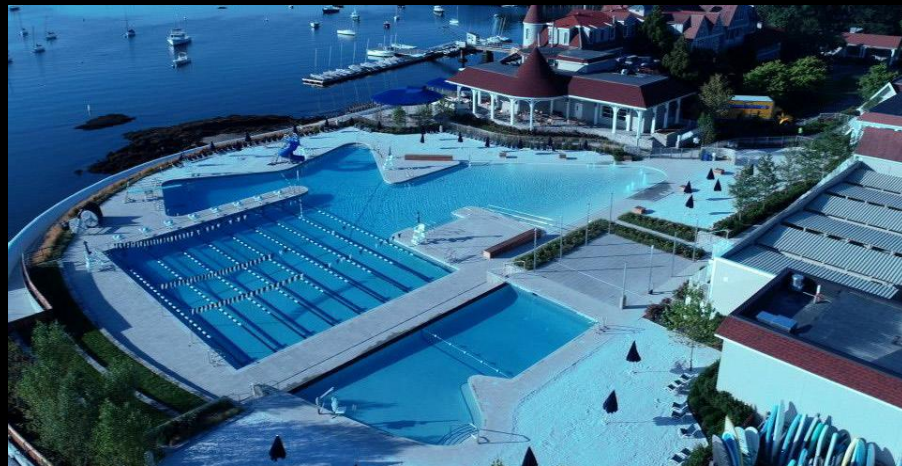
Main Line Commercial Pools, Larchmont Yacht Club
