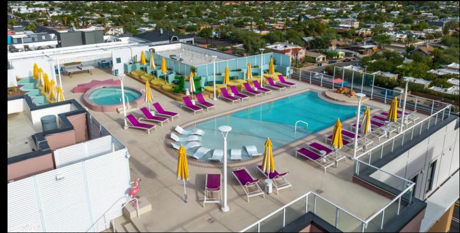
Cimarron Circle Construction, HUB Tucson
