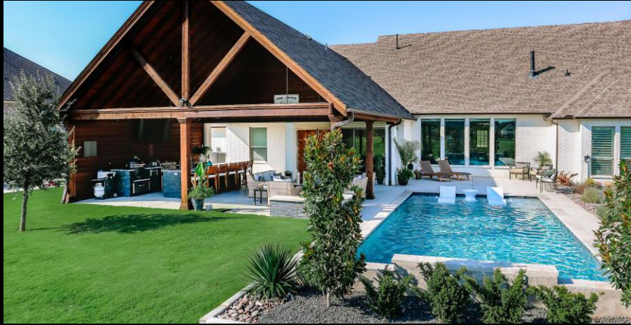
Gohlke Pools, Cates Project
