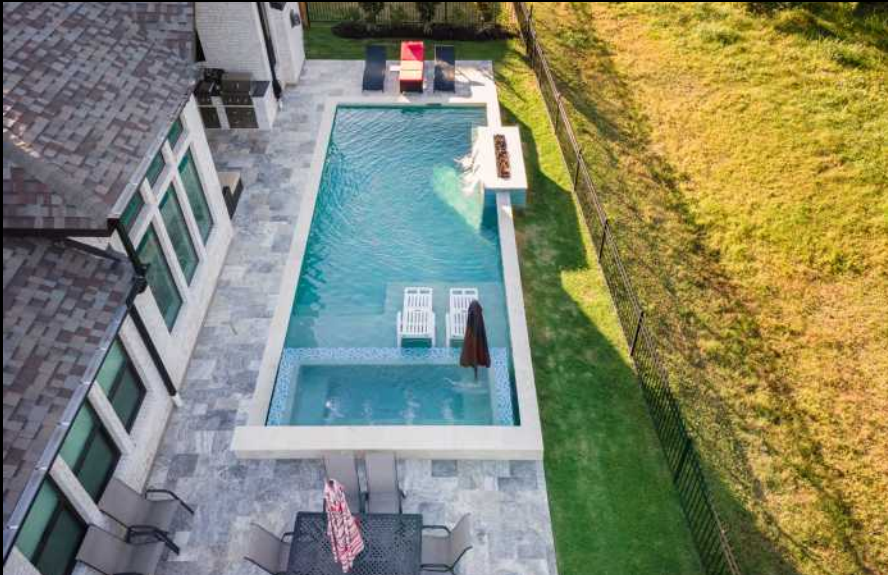
SUNSET POOLS, INC, HARRELSON PROJECT
