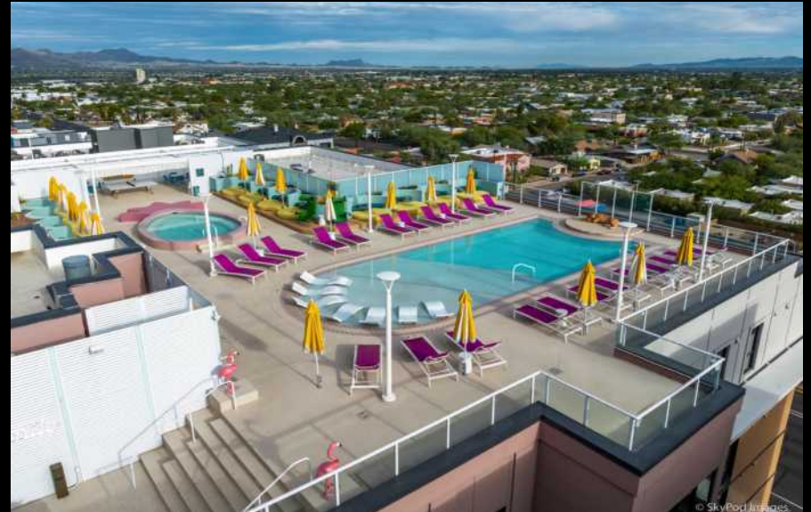
CIMARRON CIRCLE CONSTRUCTION, HUB TUCSON
