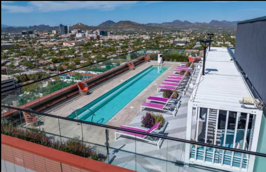
CIMARRON CIRCLE CONSTRUCTION, OLIV SPA
