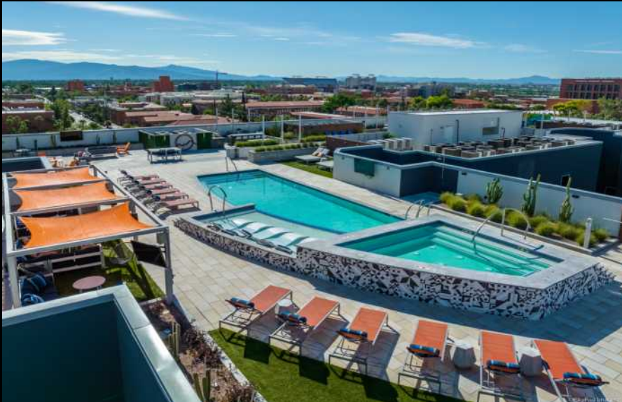
CIMARRON CIRCLE CONSTRUCTION, THE PARKER
