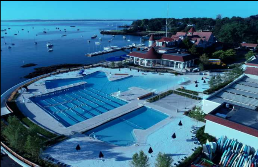
MAIN LINE COMMERCIAL POOLS, LARCHMONT YACHT CLUB
