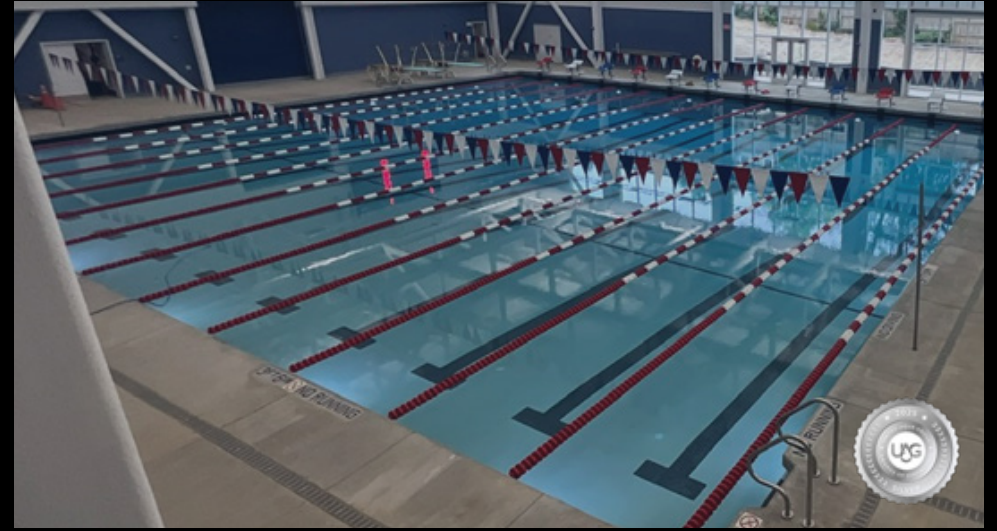
MAIN LINE COMMERCIAL POOLS - MINNIE HOWARD HIGH SCHOOL
