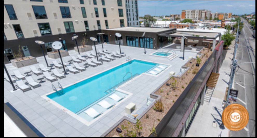
CIMARRON CIRCLE CONSTRUCTION - ARI ON 4TH
