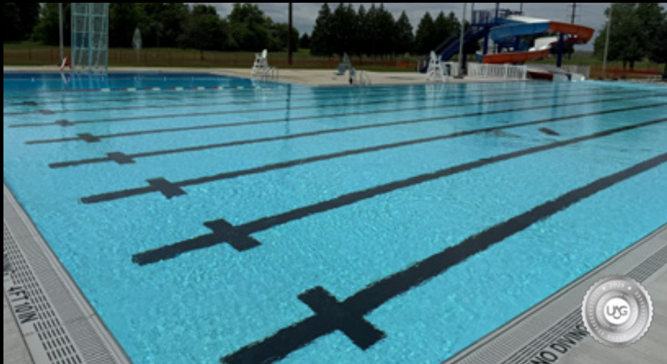
MAIN LINE COMMERCIAL POOLS - HAMPDEN TOWNSHIP COMMUNITY POOL
