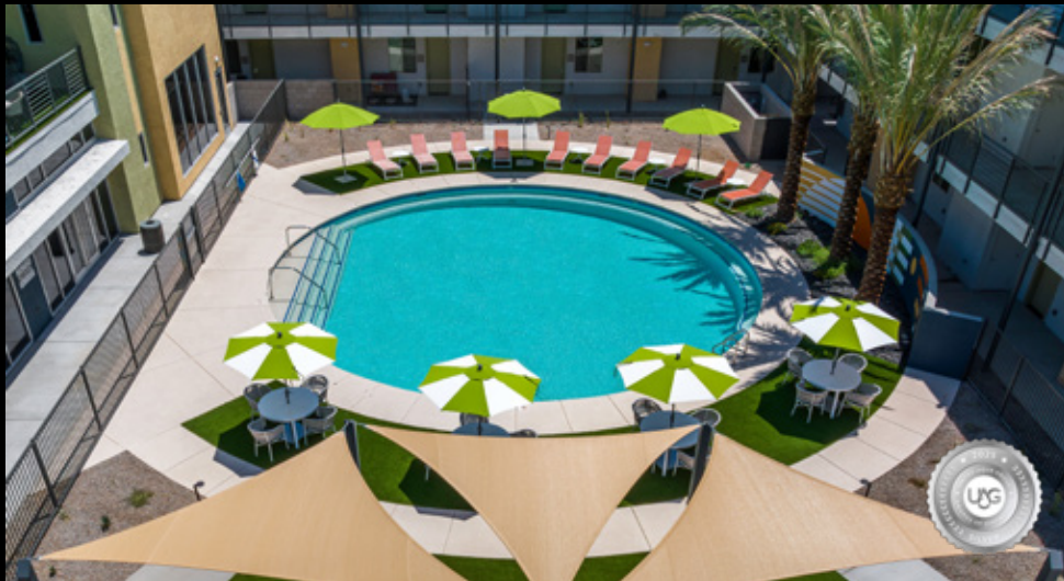
CIMARRON CIRCLE CONSTRUCTION - CABANA BRIDGES
