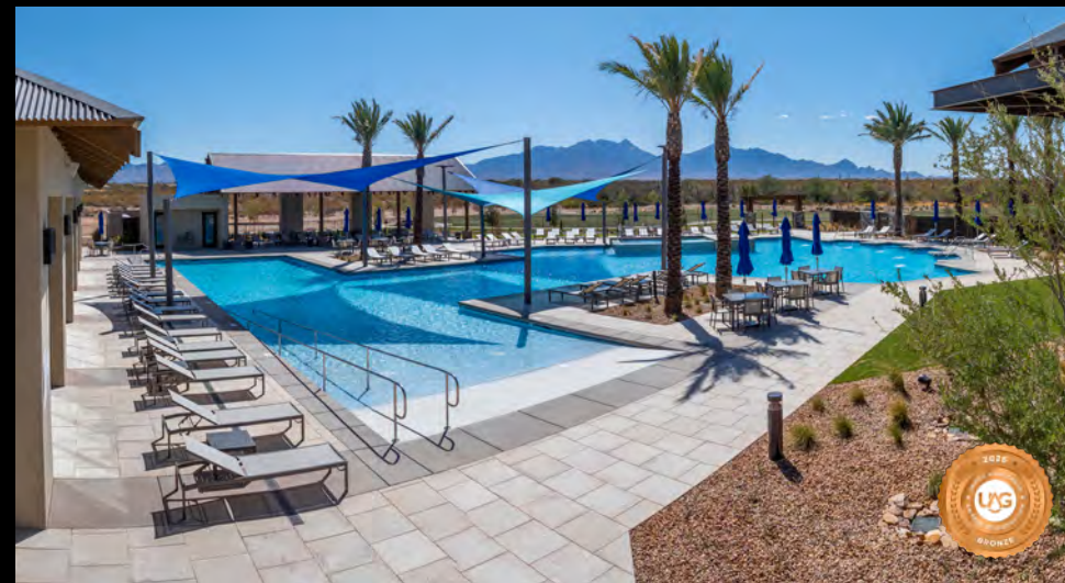
CIMARRON CIRCLE CONSTRUCTION - CANYON CLUB OUTDOOR
