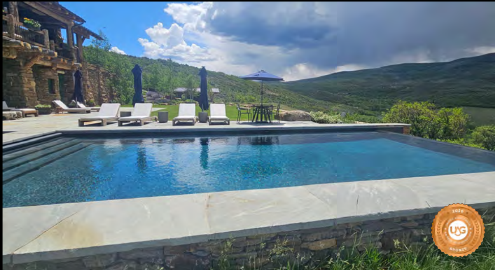
COLORADO POOL + SPA SCAPES - DEADWOOD RANCH INFINITY EDGE POOL AND SPA
